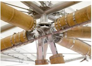
Figure 21: The use of metallic braces has become popular and added more strength to the bamboo houses
